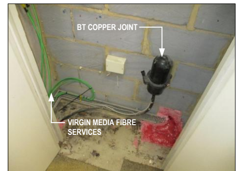
PHOTOGRAPH 9 VIEW OF EXISTING BT COPPER JOINT AND VIRGIN MEDIA SERVICES IN FIRST FLOOR RISER ACCESSED FROM STAIR WELL
