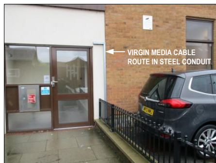
PHOTOGRAPH 11 VIEW OF VIRGIN MEDIA CABLE ROUTE FROM EXTERNAL CHAMBER TO STAIRCASE AREA ON EAST ELEVATION
