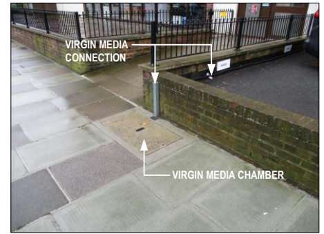
PHOTOGRAPH 6 EXISTING VIRGIN MEDIA CHAMBER AND BUILDING CONNECTION IN FOOTWAY ON ELMFIELD AVENUE OUTSIDE BUILDING
