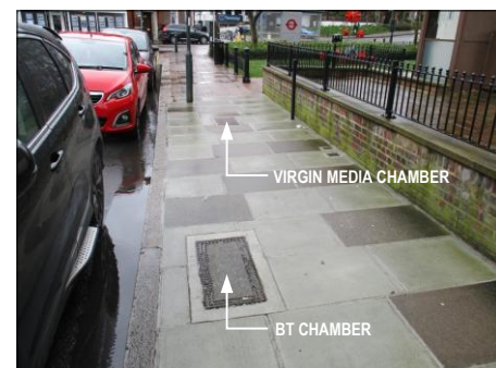
PHOTOGRAPH 3 EXISTING BT AND VIRGIN MEDIA CHAMBERS ON WEST SIDE OF ELMFIELD AVENUE OUTSIDE BUILDING
