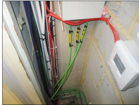
PHOTOGRAPH 14 TYPICAL VIEW OF EXISTING TELECOMS SERVICES IN RISER ON FIRST FLOOR
