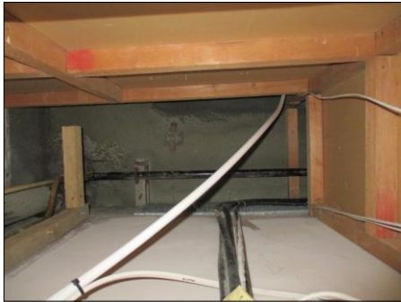
PHOTOGRAPH 13 VIEW OF BT COPPER AND FIBRE SERVICES FROM GROUND FLOOR INTAKE LOCATION TO FIRST FLOOR CEILING LEVEL
